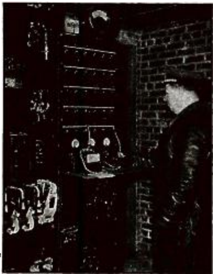
Control panel for the new U.S. Navy blind-landing system. Current supplied by a 500-cycle motor-generator is fed through this panel to the buried cables which set up the magnetic beam (which has a range of 9,000 ft.).
